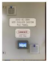
temperatures, flow and pressures and adjusts the response accordingly to maintain continuous supply of chilled water and maintain positive pressure operating environment within the enclosure. The control system can be manually operated within the VSD chiller enclosure via the HMI but is primarily linked back to the Howden switch room via ethernet.
