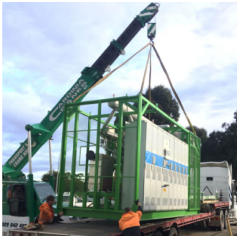
ORC Generator ready for shipment from gTET
