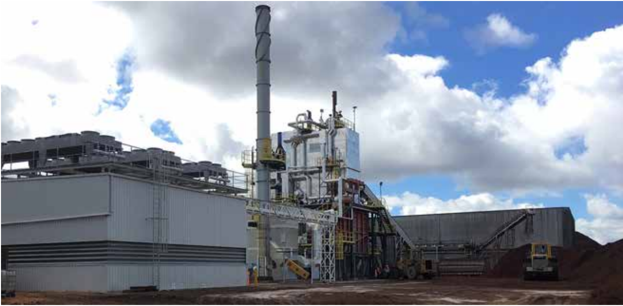
Biomass power station, ORC generator building foreground with the biomass boiler in the far ground and grape marc fuel mound on the right
