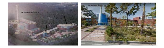
The incinerator/biomass boiler produces approximately 9T/h steam at about 15bar.
